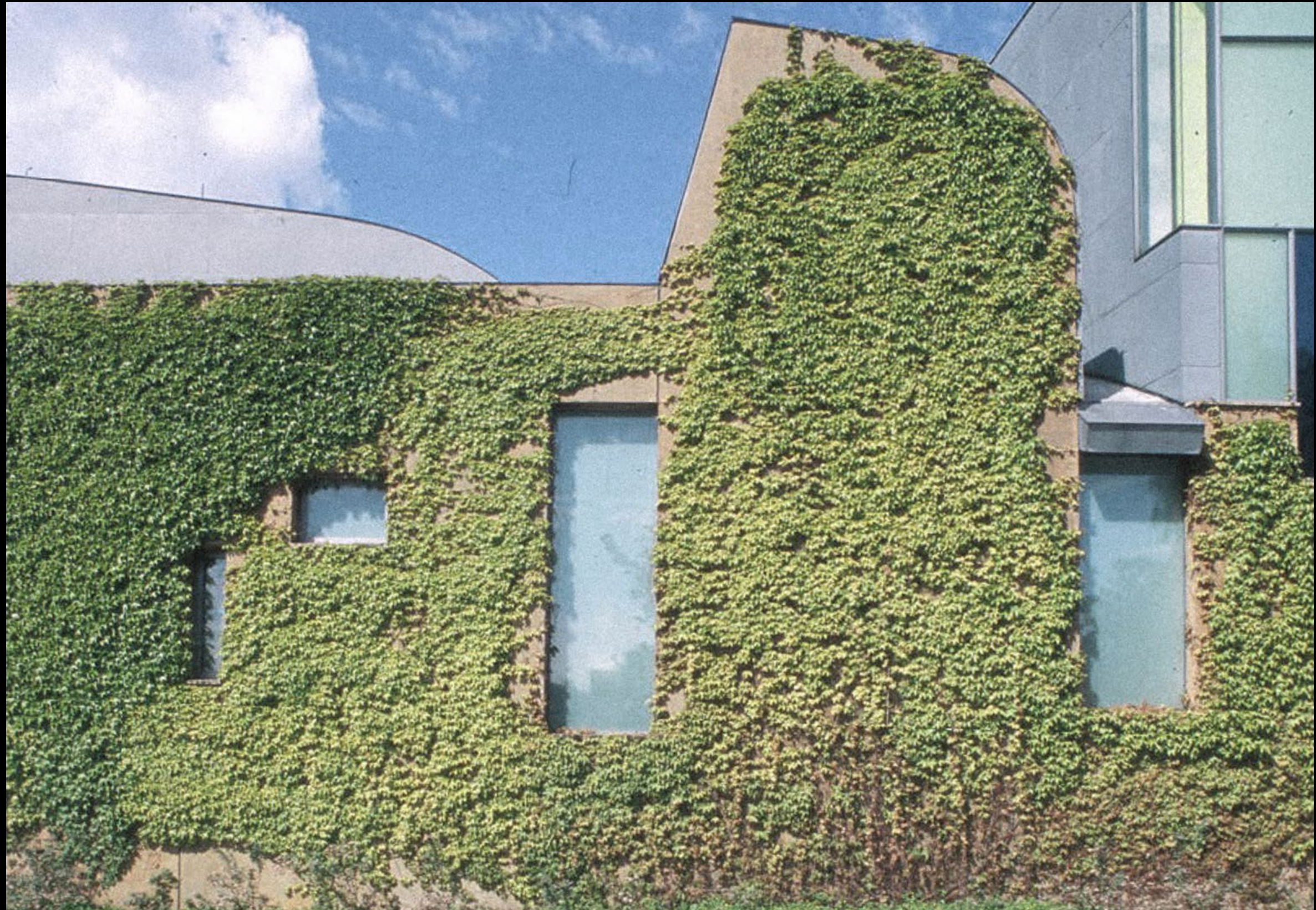
SEATTLE, WA ST. IGNATIUS CHAPEL 1997
