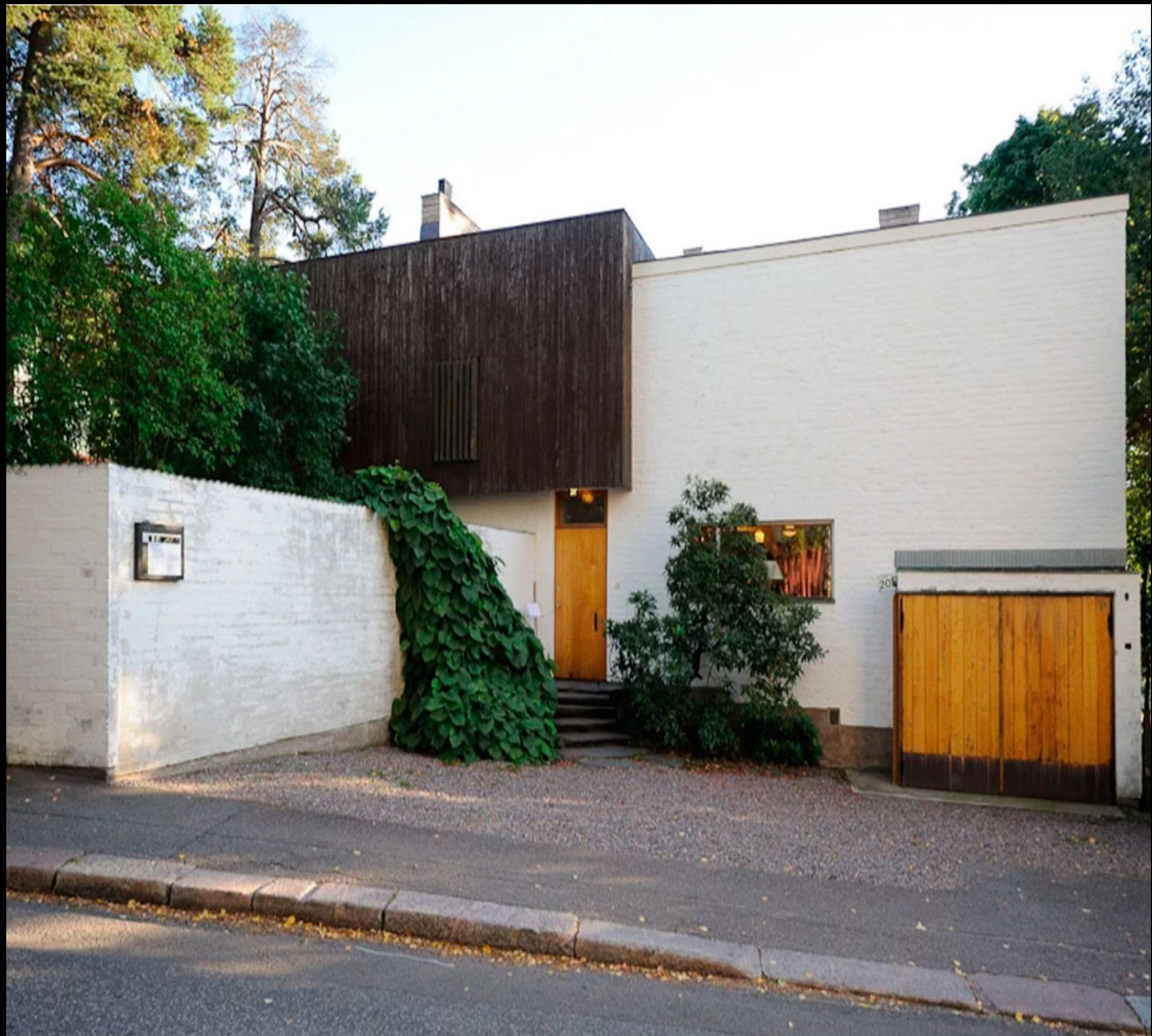
Aalto's Home Helsinki, Finland Alvar Aalto 1936
